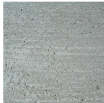
Insitu Broomed Concrete Paving PEDESTRIAN PAVING
