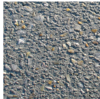
Insitu Exposed Aggregate Concrete PEDESTRIAN PAVING
