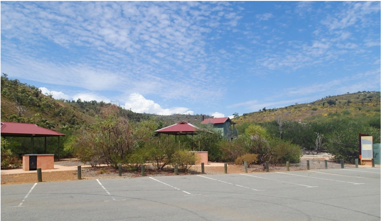
Plate 20: Barbeques, Shelter and Toilet facilities in Honeyeater Hollow, part of New Visitor Experience
