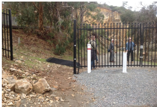
Plate 25: Broken Gates leading to Barrington Quarry
