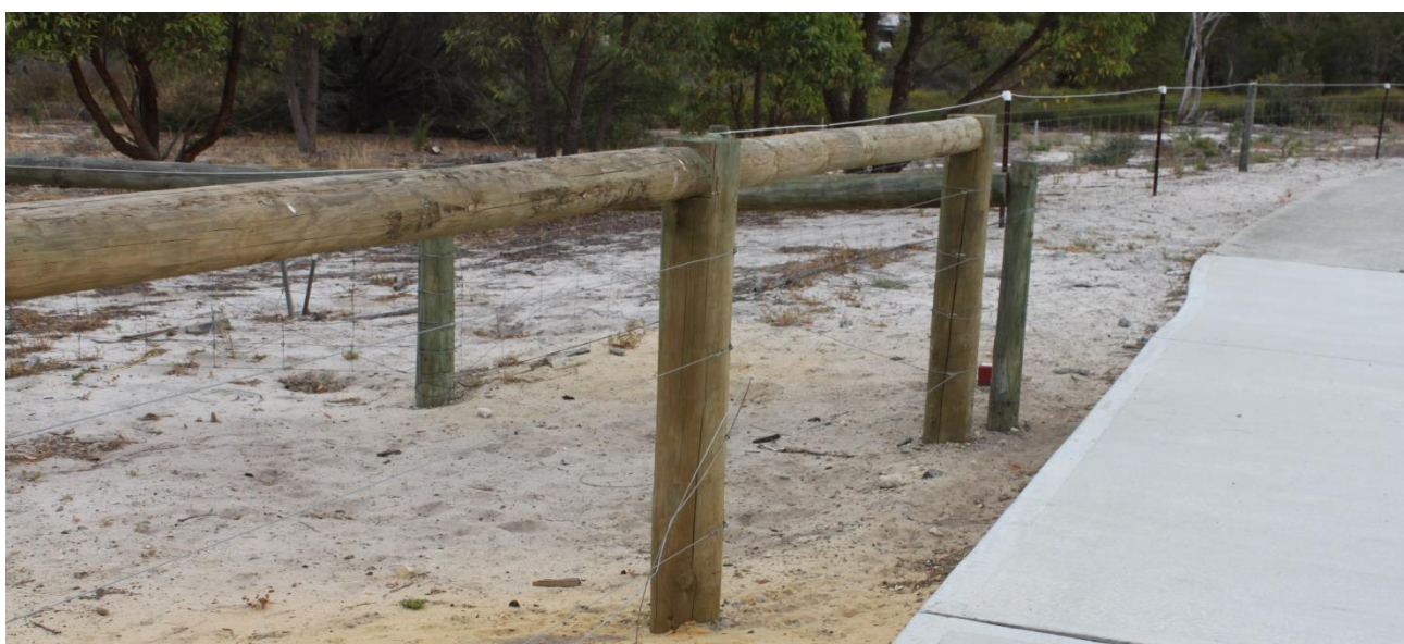
Figure 8: Post and rail fence
