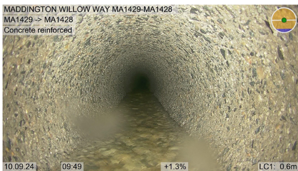
MA1429-MA1428_8d249dfc-b3f4-4b81-8e0f-8882d939a1de_20240910_094959_338.jpg, 00:01:11, 0.60 Surface damage concrete, spalling of the concrete conduit including localised chipping from 12 o'clock to 12 o'clock, Start
