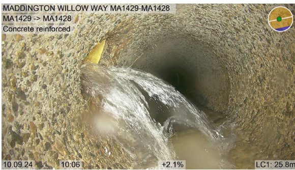
MA1429-MA1428_e49bd966-94cd-45a2-9ad9-66848dfed0ea_20240910_100641_616.jpg, 00:13:44, 25.80 Connection, unlined, connection appears to be open, Height/Diameter (mm): 90 at 10 o'clock
