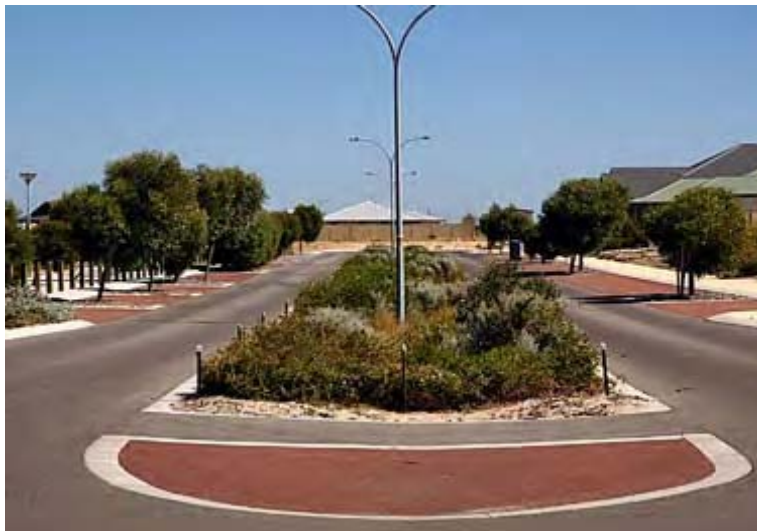
Median Swale Stormwater Manual Western Australia
