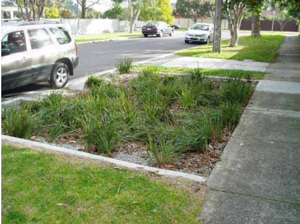
Roadside Bio-Retention and Filtration Pocket Picture from Review of Street Scale WSUD in Melbourne - Study and Findings
