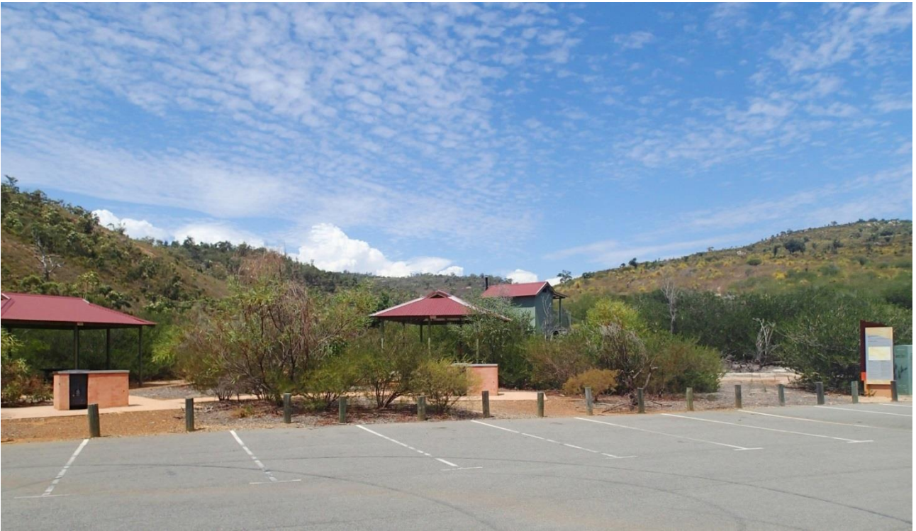
Plate 20: Barbeques, Shelter and Toilet facilities in Honeyeater Hollow, part of New Visitor Experience
