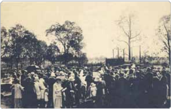
Laying of foundation stone at St Luke's Church, 1926. Courtesy City of Gosnells Museum.
