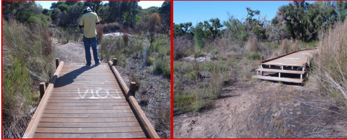
Figure 24: Boardwalk Terminating at Steps Providing Direct Access to Wetland
