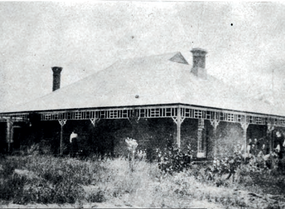
Image: Emma Wilkinson on the porch of Wilkinson Homestead c1918.
